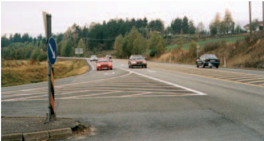
Rv 35 Vikersund. A large vehicle in the turning lane can hide a motorcyclist in the through lane.
