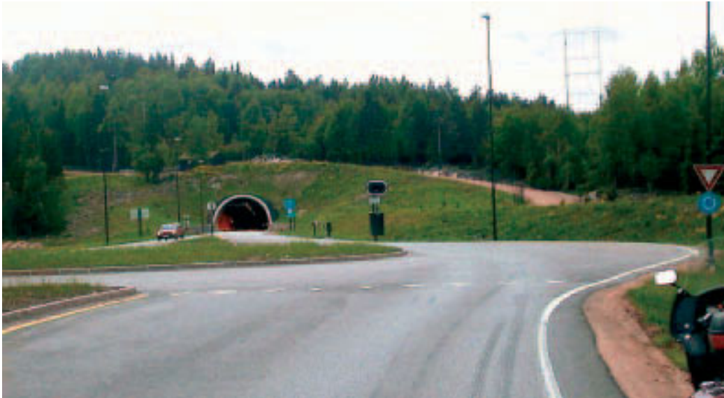
On the Oslofjord connection through Røyken and Hurum, the roundabouts are not easily detected and have a wide approach.
