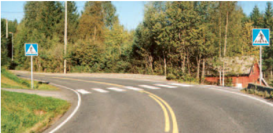
Pedestrian crossing on a curve is a poor solution both because motorcyclists may skid on the slippery markings and because the visibility relative to crossing pedestrians and cyclists is poor.
